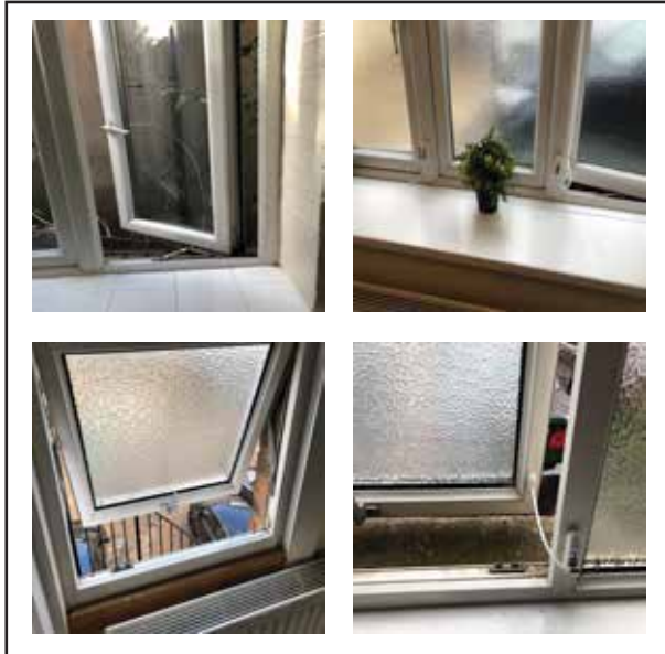
All windows are installed with safety stoppers.
