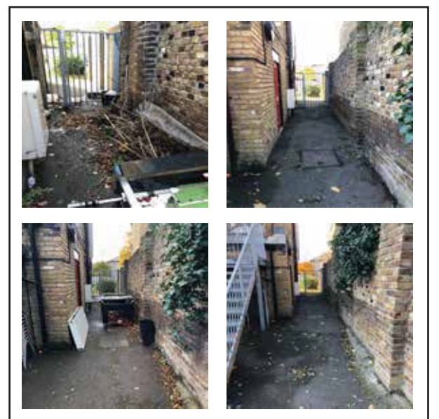
ALL fire exit routes are clear of any obstructions and hazards.
